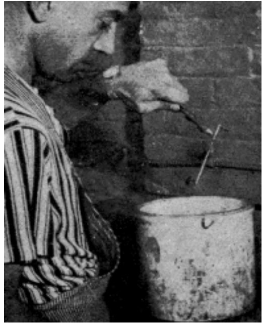
To remove silver soldering flux, use a pickle.
